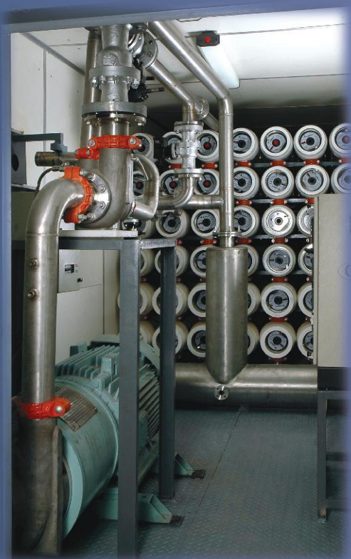
Internal View of Containerized Desalination Plant
