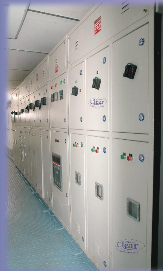
VFD & Electrical Panel - Containerized.
